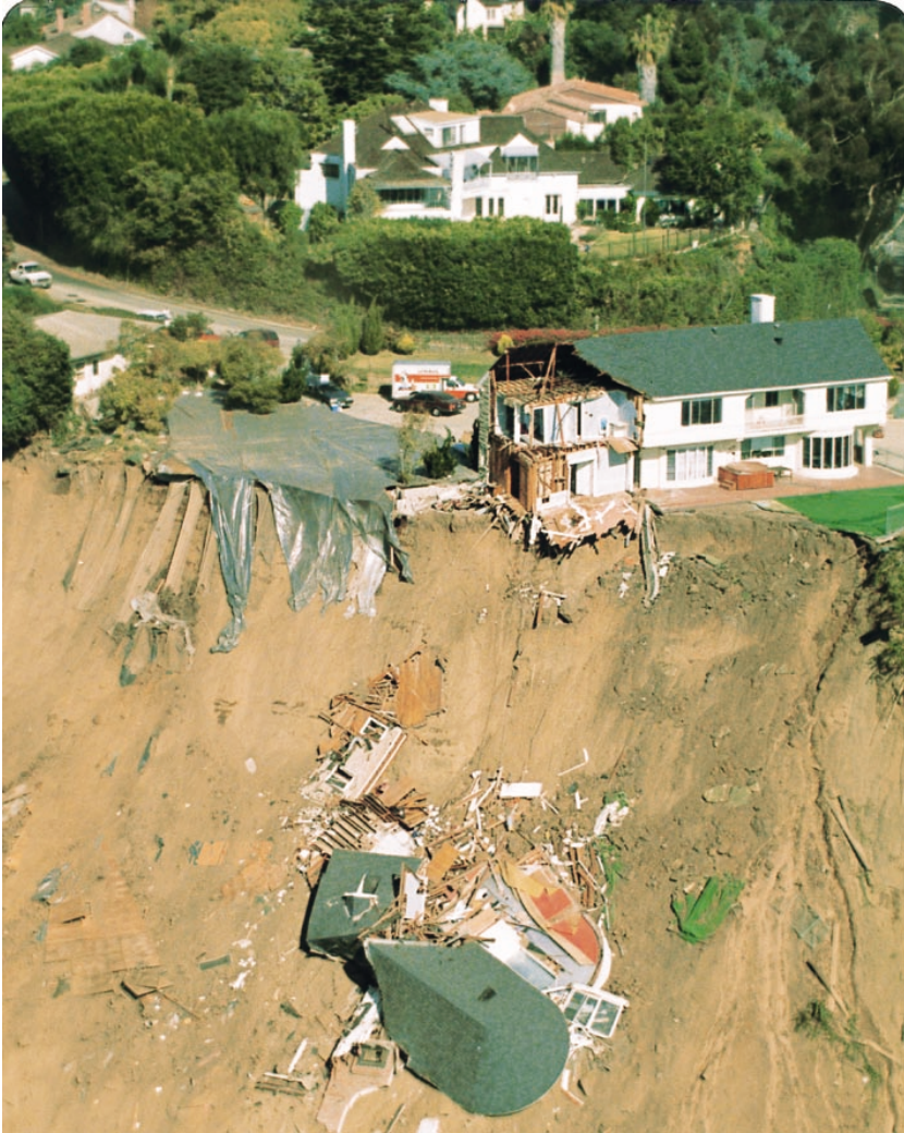
This home in the Pacific Palisades section of Los Angeles was destroyed in the 1994 Northridge earthquake. Photograph courtesy of AP/Wide World Photos.
