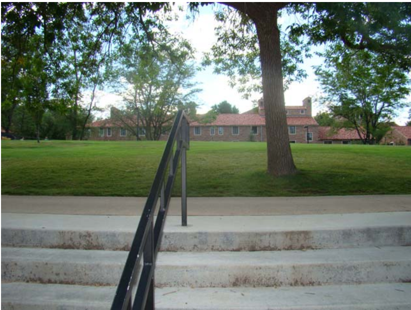
Patrons can exit on the west stairway and onto the grass field in the case of an emergency
