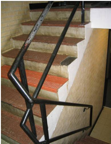
Non-Compliant Guardrails
