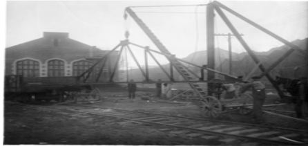
Power House Circa 1910
