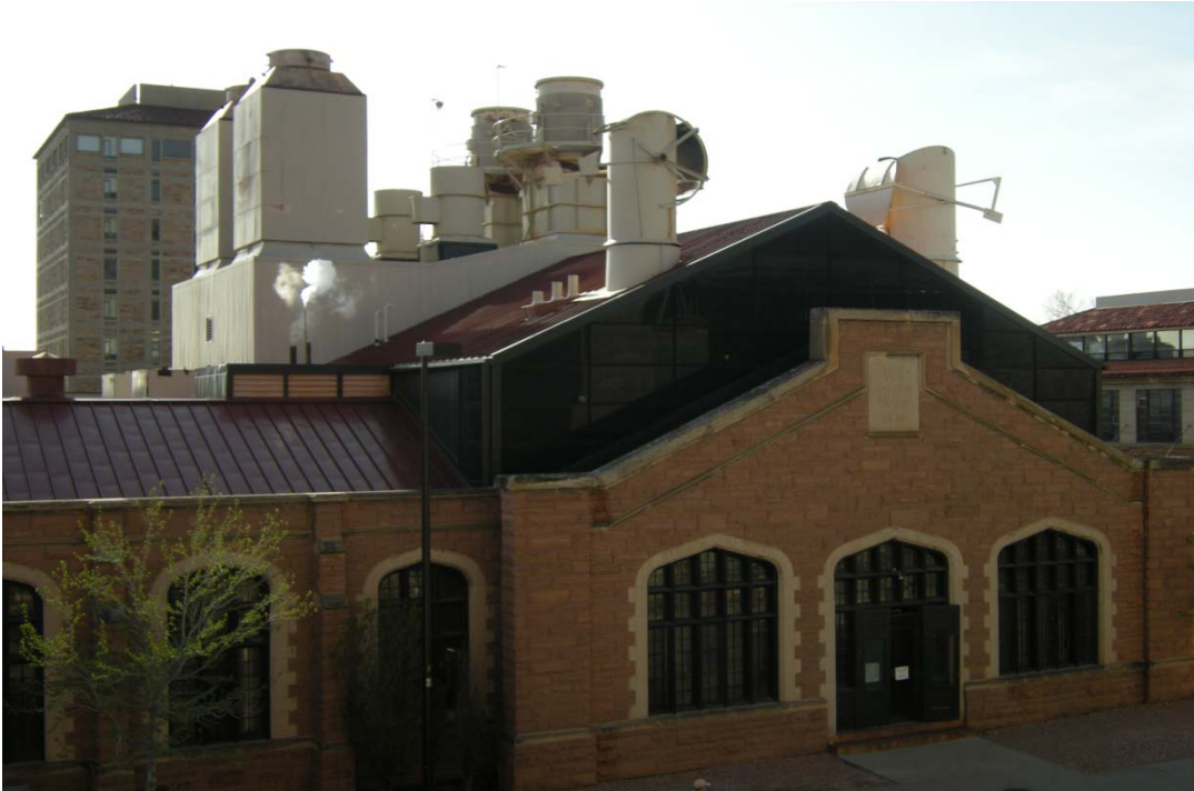
Power House University of Colorado Boulder 2009
