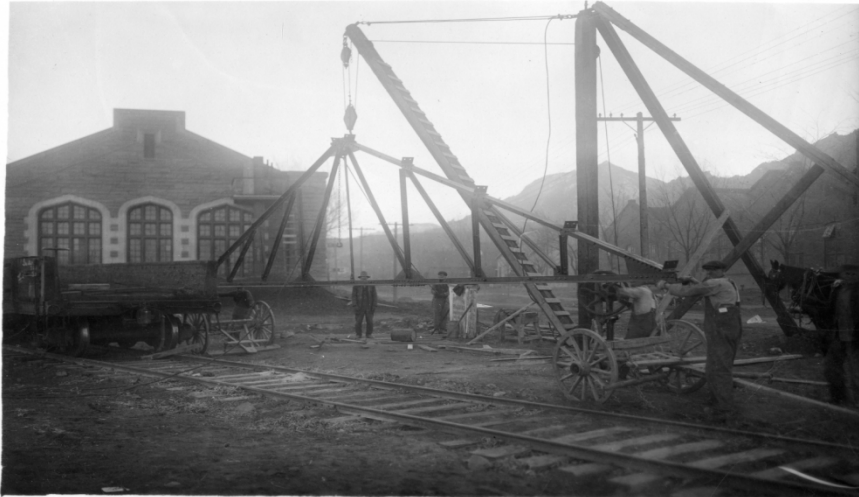
Power House Circa 1910
