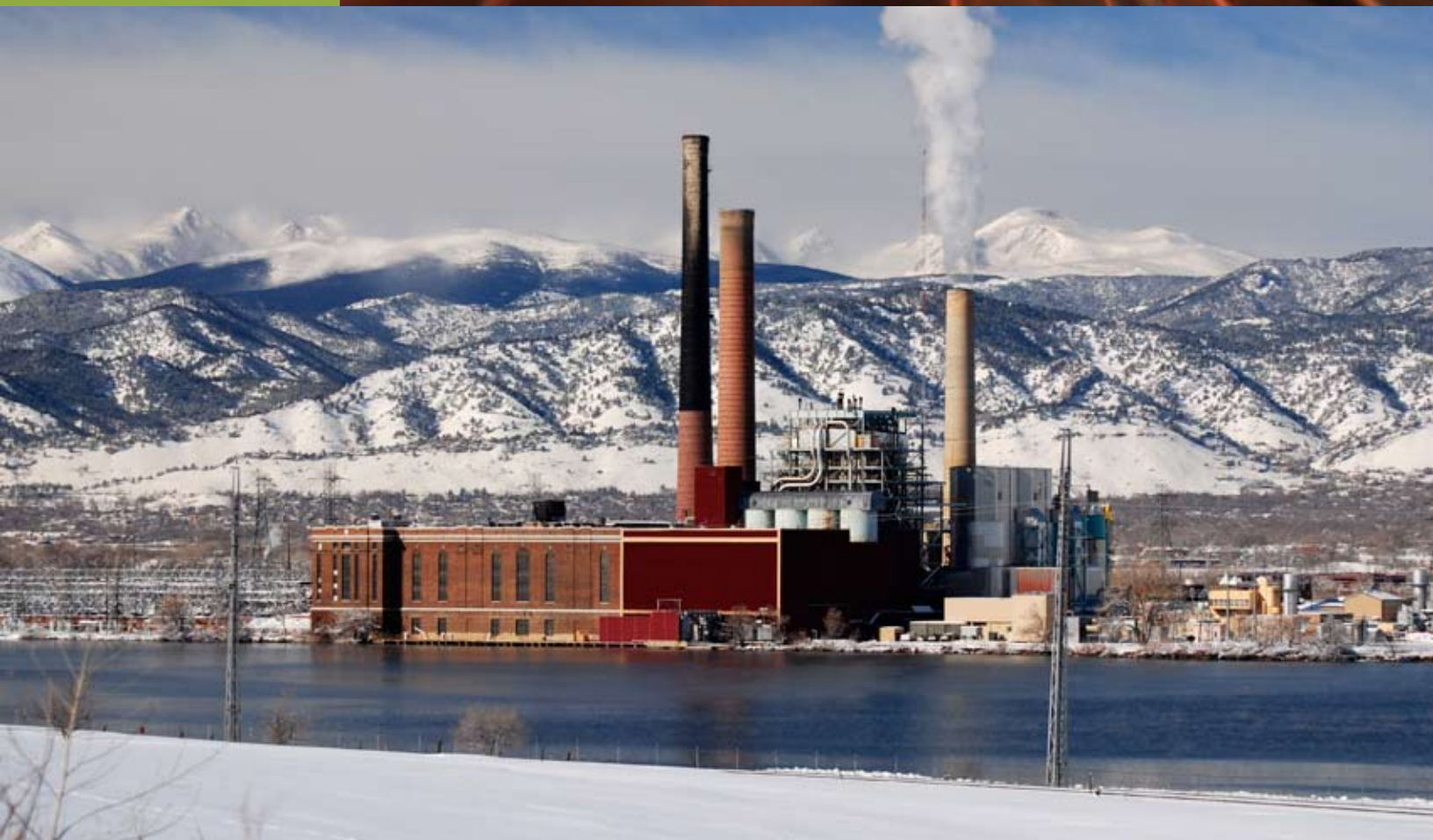
Professors Rich Noble and Doug Gin collaborate with ION Engineering to efficiently remove CO 2 from fossil fuel power plants such as the Valmont Power Plant in Boulder, pictured above.
