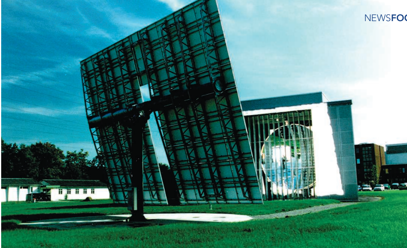
Mining the sun. This solar thermochemical fuels setup in Switzerland focuses sunlight on a reactor ( right ) that splits either water or \text{CO}_2 with the help of a zinc-based catalyst.
