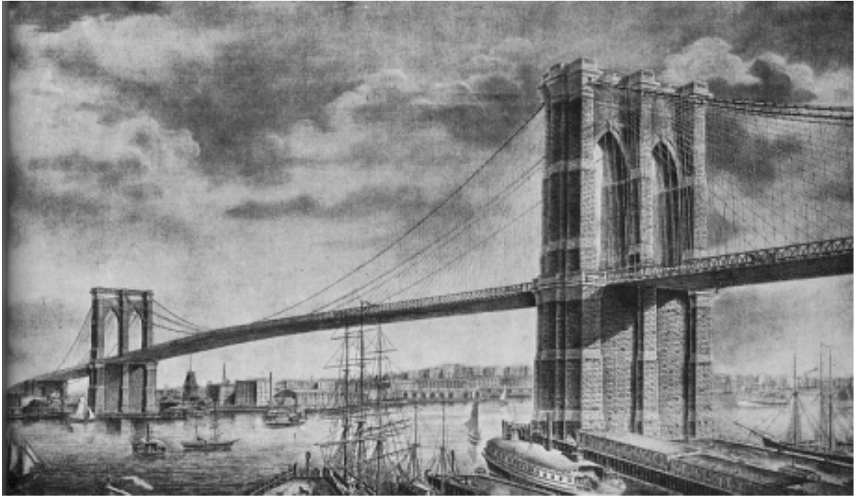
Figure 3.1. The Brooklyn Bridge in 1876, drawn by F. Hildebrand for the Library of Congress.
